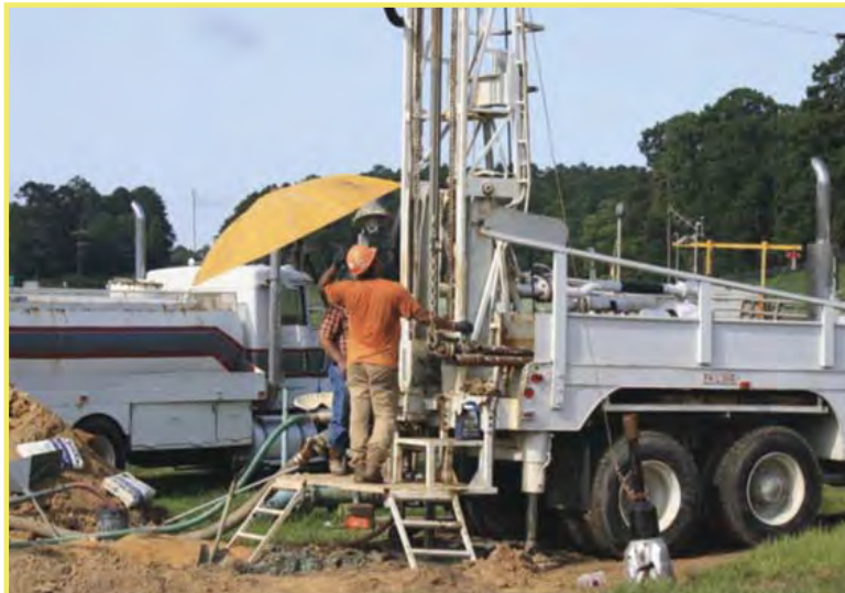
Drilling New Relief Well Near the Powerhouse
