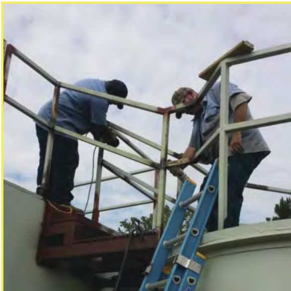
Assembling Frontier Park Wastewater Treatment Plant
