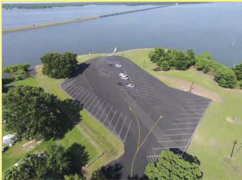
New Surface on the Farm-to-Market Highway 17 Boat Ramp
