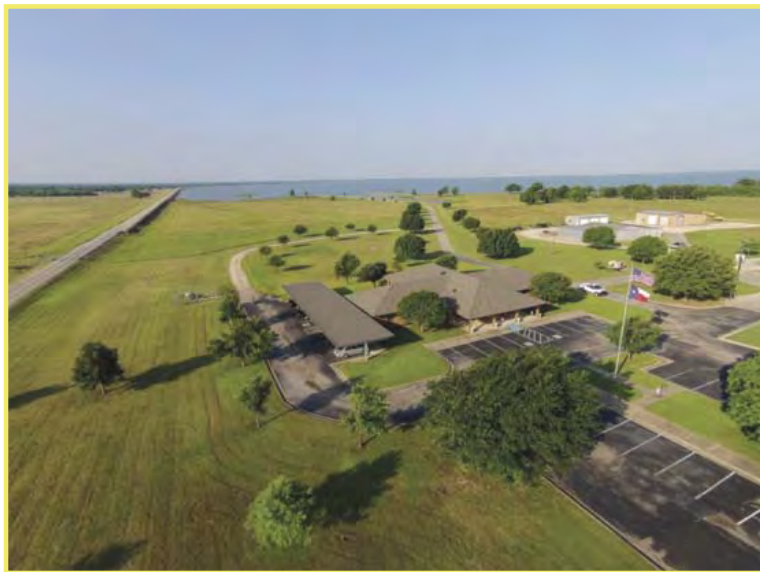
Iron Bridge Division Offices
