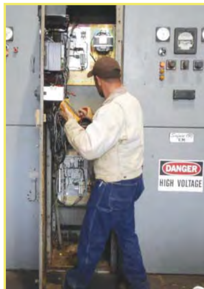
Pump Control System Maintenance
