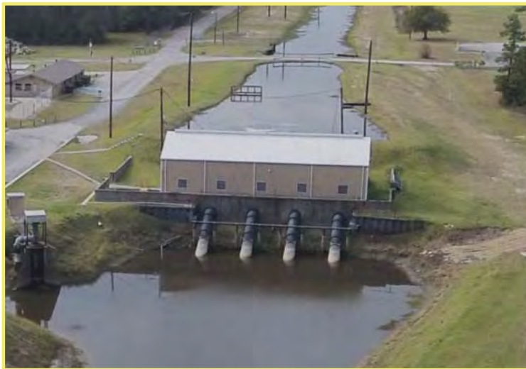
Gulf Coast Division Pumping Plant
