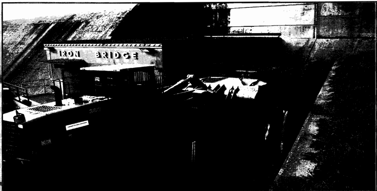
Installing the new 80 kW Emergency Generator at the Spillway
