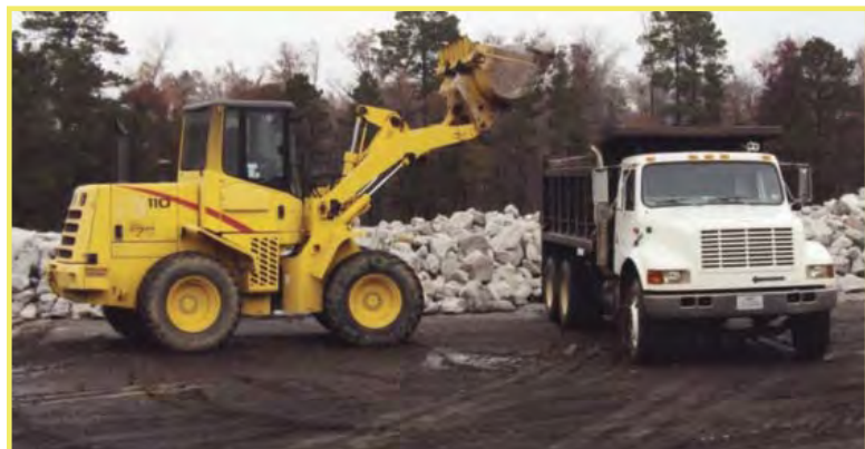
Loading Rip-Rap for Shoreline Management
