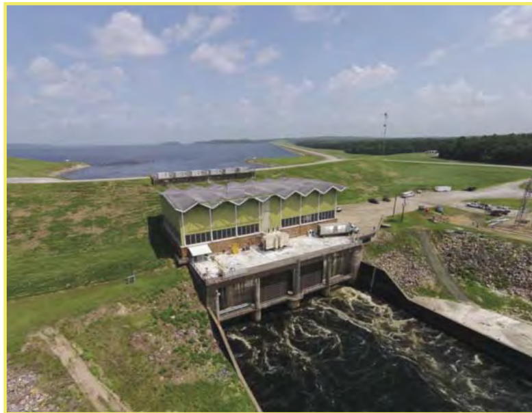
Toledo Bend Dam and Powerhouse
