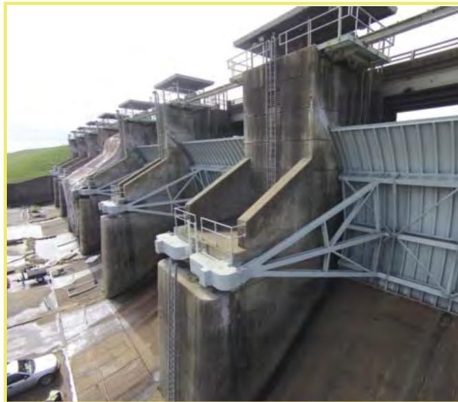
Gate Refurbishment at Toledo Bend Spillway
