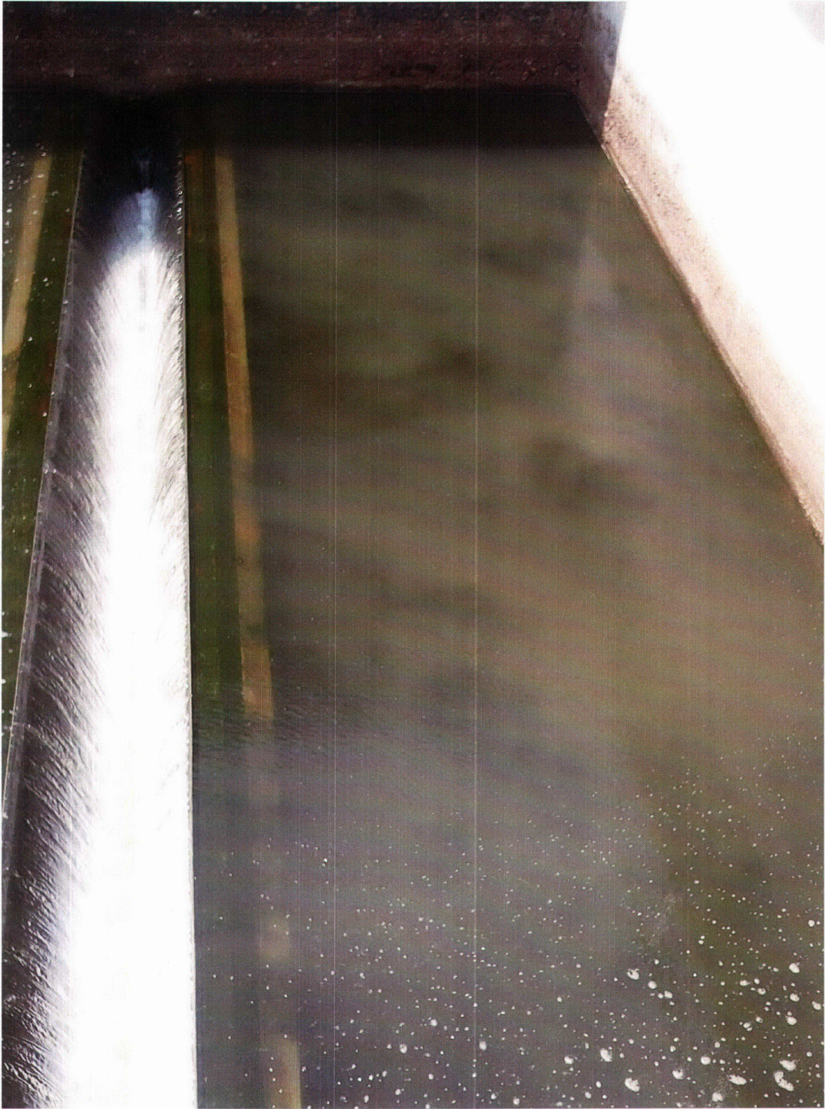
Figure 2.1 - Cloudy water observed during backwash to waste operation. After 20 minutes of combined air/water backwash
