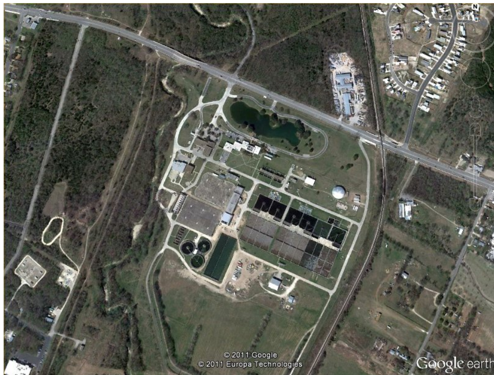
Figure 2-1 – Aerial Photo of the Walnut Creek WWTP Site
