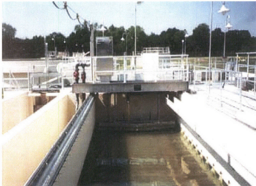
Figure TM2-9 - Automatic Traveling Bridge Filter System
