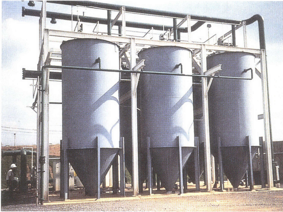
Figure TM2-12 - Upflow Filtration System
