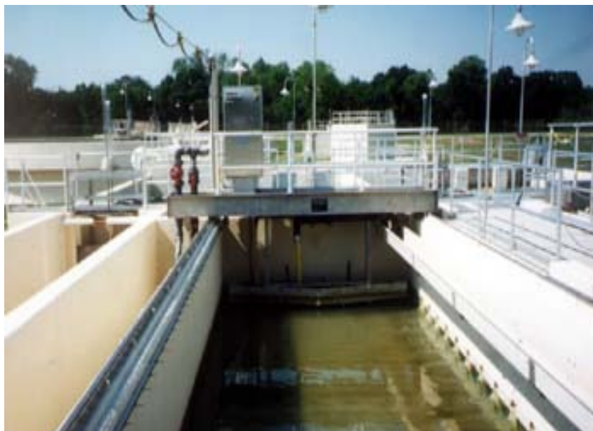
Figure TM2-9 - Automatic Traveling Bridge Filter System
