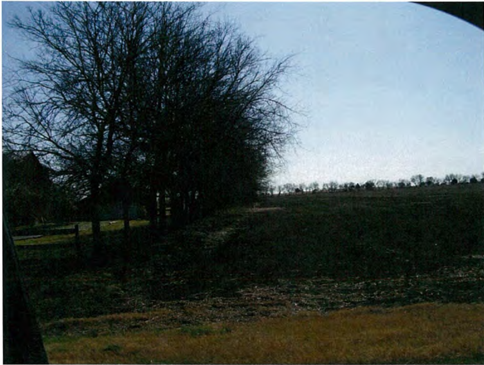
P21. Road drainage off of FM 1552 looking north. The drainage had no identifiable OHWM.
