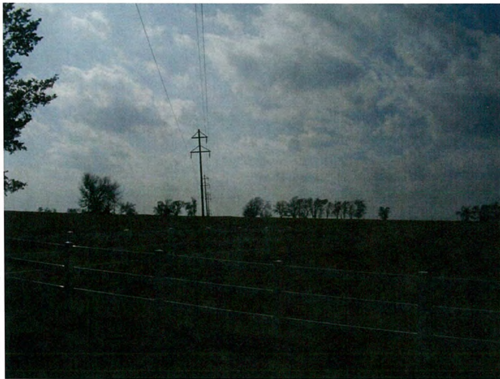
P58. Pipeline ROW following a power line ROW, looking southwest.
