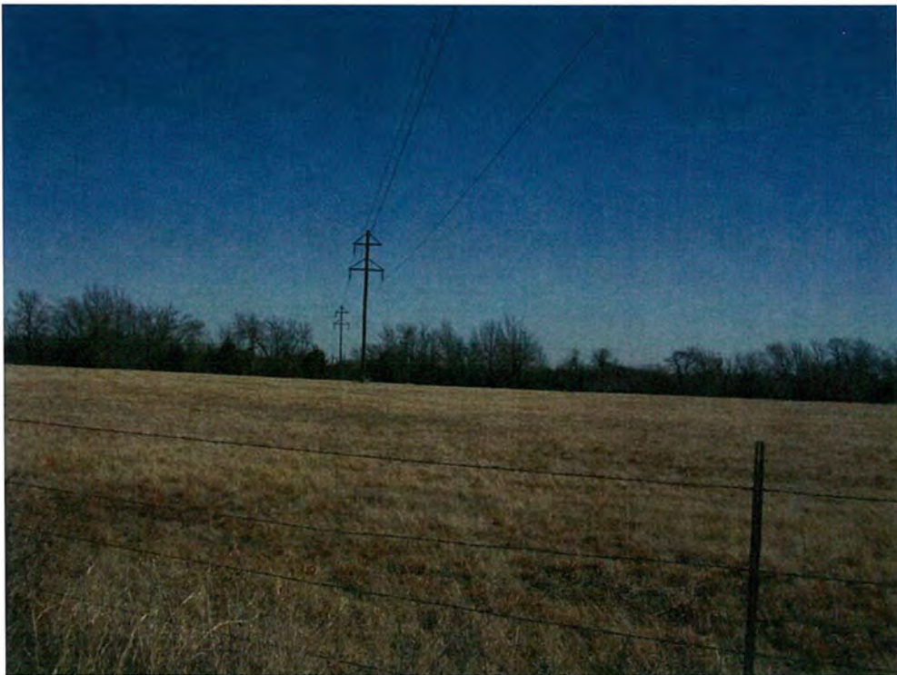
P38. Pipeline ROW following a power line ROW, looking northeast.
