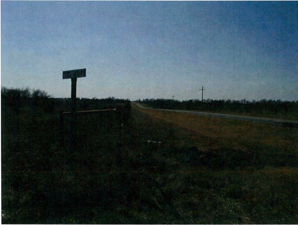
P25. State Highway 78 and County Road 4815 intersection, looking southwest.
