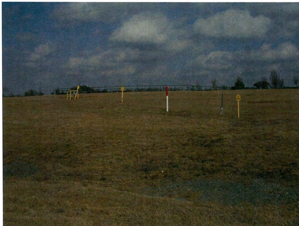
P60. Pipeline ROW following a gas pipeline ROW, looking northeast.
