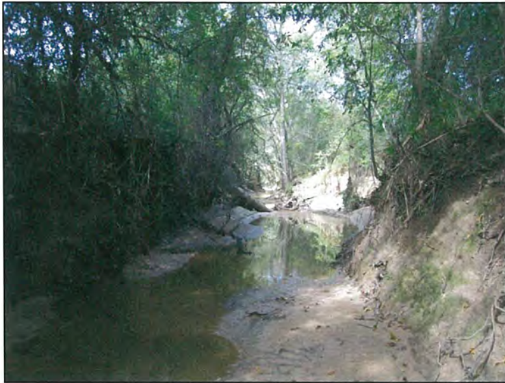
Figure 5.42: Typical View of Sandy Creek with vertical side slopes.
