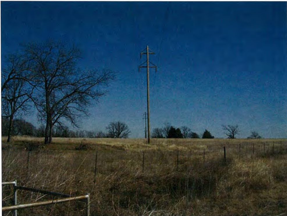
P46. Pipeline ROW following a power line ROW, looking northeast.
