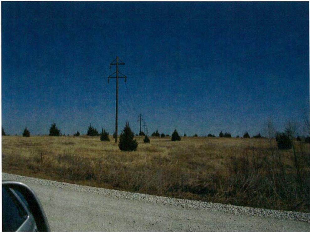
P51. Pipeline ROW following a power line ROW, looking northeast.
