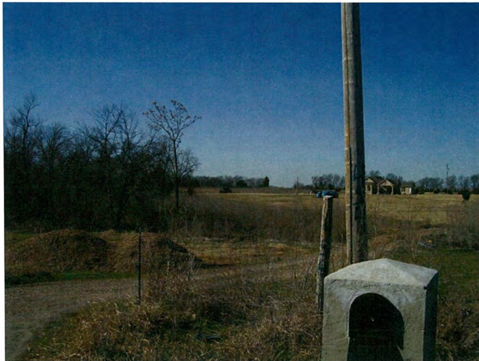
P32. Culverted crossing of an Unnamed tributary to South Sulfur River, looking west.
