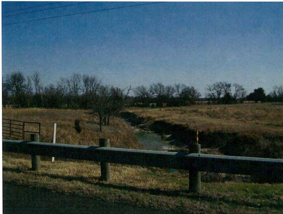
P30. Drainage to South Sulfur River, looking downstream east.
