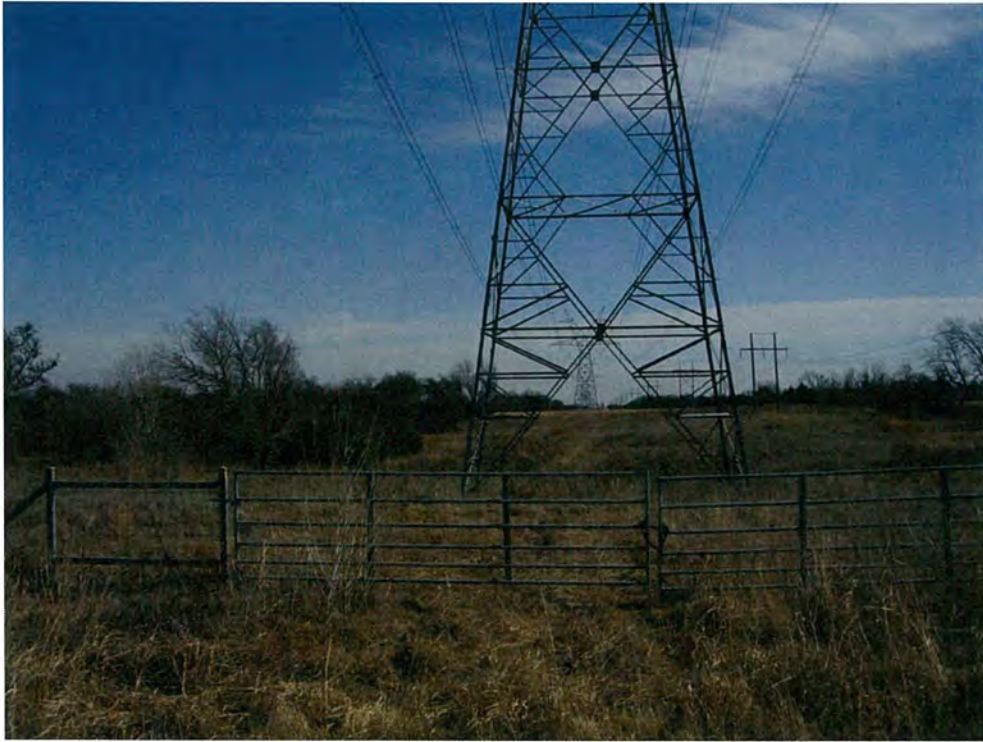
P5. Powerline right of way where pipeline would follow, looking east.
