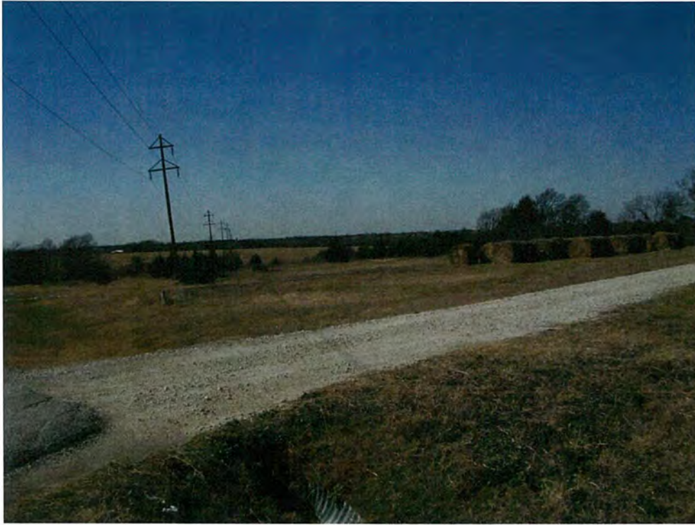
P43. Pipe crossing at FM 881 and County Road 5020 intersection, looking northeast.
