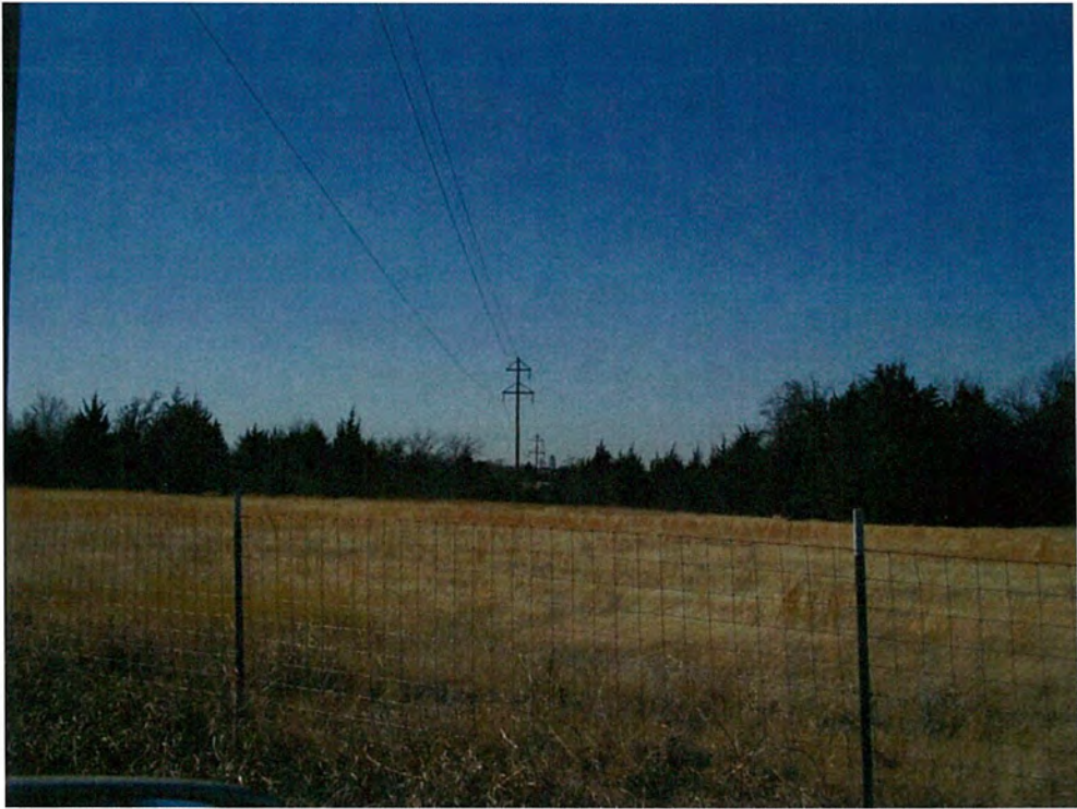
P39. Pipeline ROW following a power line ROW, looking southwest.
