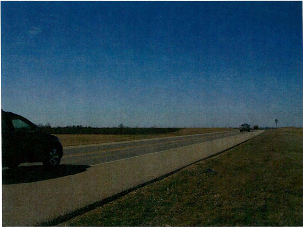
P8. Pipeline ROW at crossing of U.S. Highway 82, looking east.
