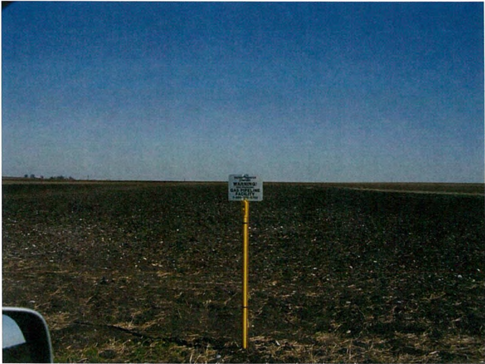
P15. Pipeline crossing of County Road 3120, looking east at gas pipeline marker.
