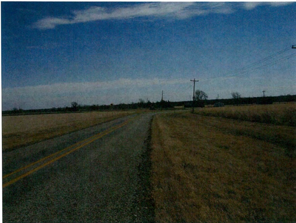
P10. Pipeline ROW at FM 1743 crossing, looking east.
