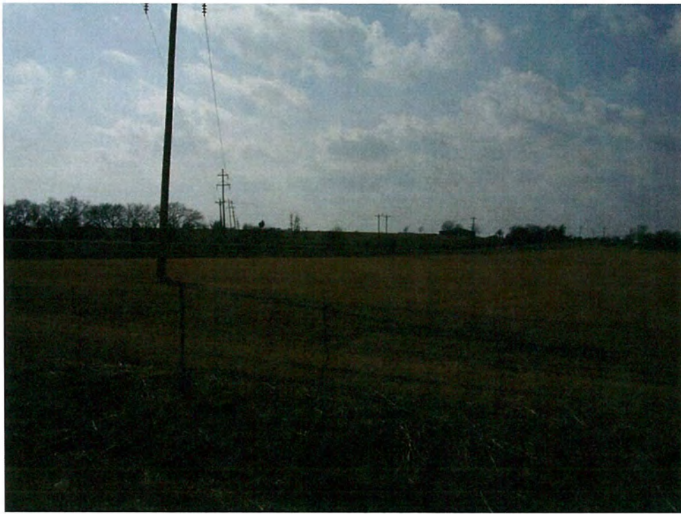
P56. Pipeline ROW following a power line ROW, looking southwest.
