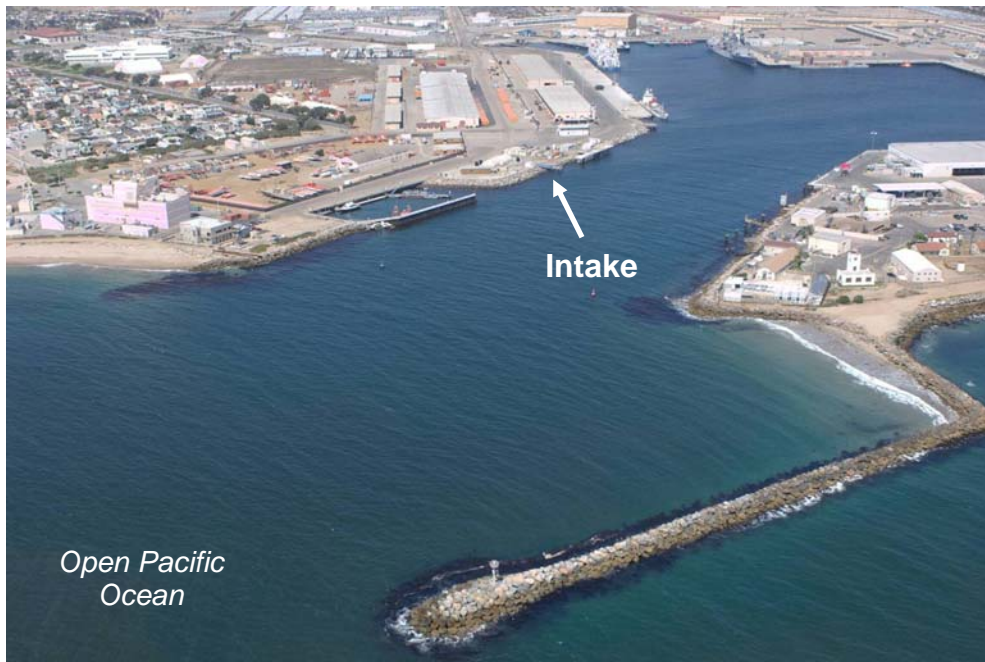
Figure 3.1 Raw water intake at Port Hueneme
